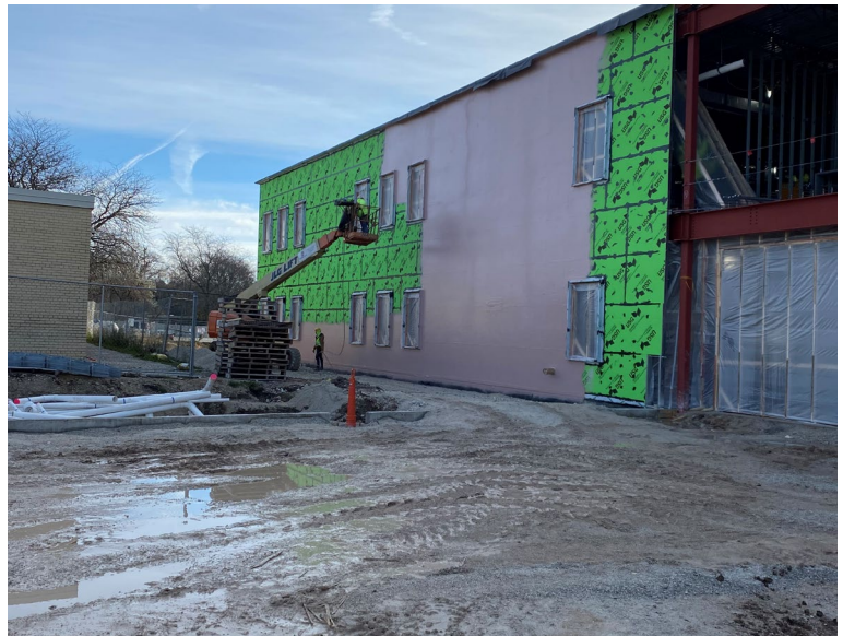
Spraying air vapor barrier on the exterior of Area C.
