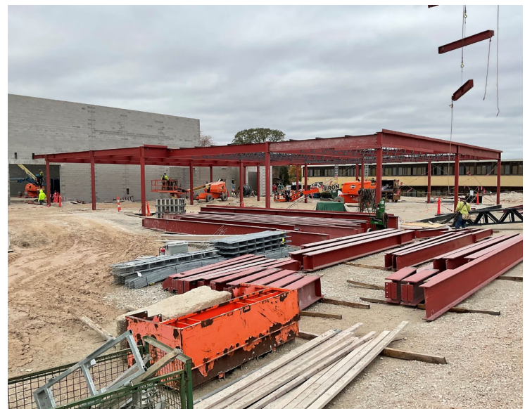
Setting the structural steel in Area A.
