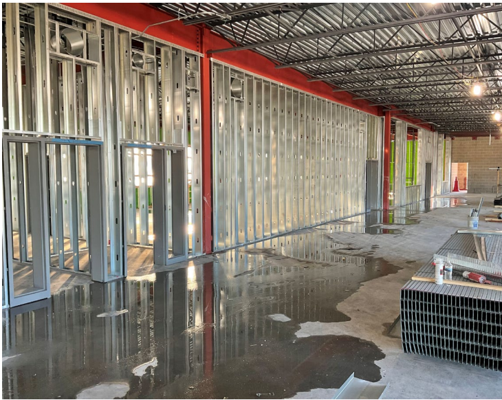
Installing interior metal studs on second floor Area C.
